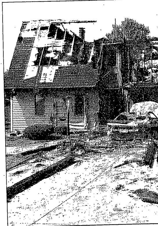
This triplex in Wilkshire Hills sustained heavy d
